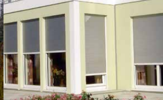
Time-controlled switching – „good morning“ on the dot
